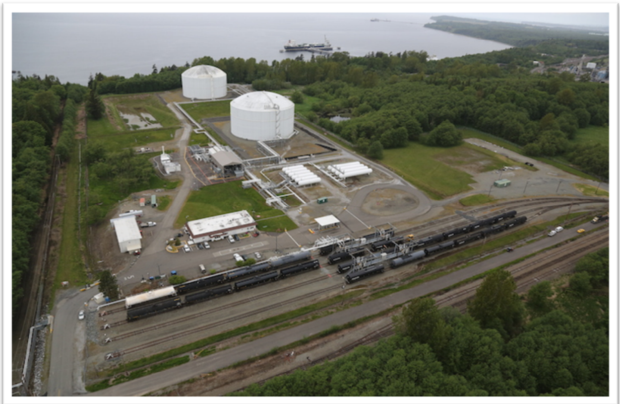
Figure 5 - Aerial view looking west of Ferndale Propane Export Facility, Washington
